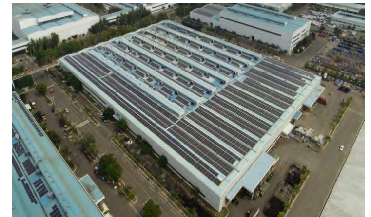
Photovoltaic power generation in Hyundai’s plant in India
